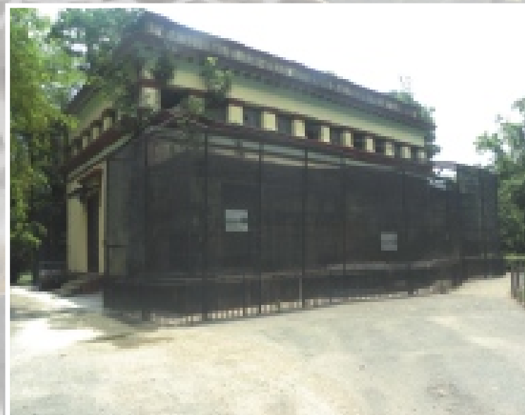
Gubbay House: The Gubbay House was built to commemorate the name of Mr. Ellias Gubbay. The enclosure is an oblong brick-made edifice measuring 50 feet long by 30 feet broad by 22 feet high with an arched roof. Previously it was the house of Apes and Monkeys. At present it is renovated for Nocturnal House.
